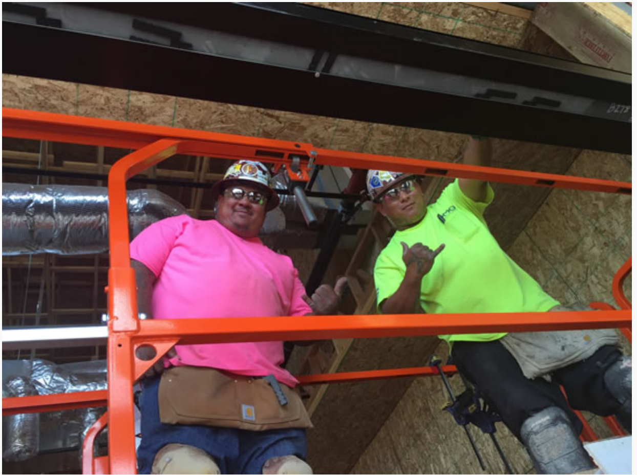
Shown here are 2 union certified glaziers at work on the project. Giroux Glass, Inc. employs only union-certified glaziers. Shown here are Jonathan "Junior" Perez and Kawelo McKeague at work.
