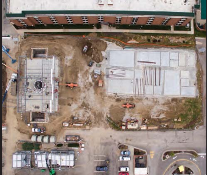
Lithko Contracting LLC (No. 42) did all the concrete work, including a base that was 50% below grade as well as 58-ft-tall towers at each end of the tilt-up concrete structure, for the i-Fly Indoor Skydiving Facility in Overland Park, Kan.
